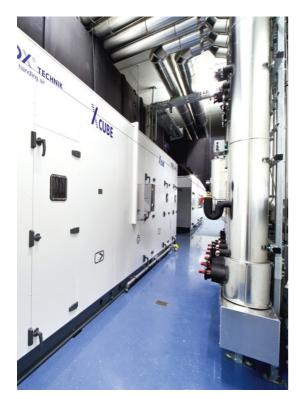
In highly sensitive areas, more than anywhere else, an air handling unit must meet particularly stringent requirements. The TROX X-CUBE is an air handling unit with unlimited configuration options of which even the basic version has set a new standard for hygiene and quality. It takes only a few measures to arrive from the top-of-class construction for various applications to an air handling unit which meets particularly high hygiene requirements:
