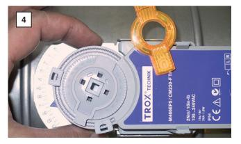
Set  $\dot{V}_{min}$  or  $\dot{V}_{max}$  on the rotary knob; reattach the mechanical limiters in the corresponding positions.
